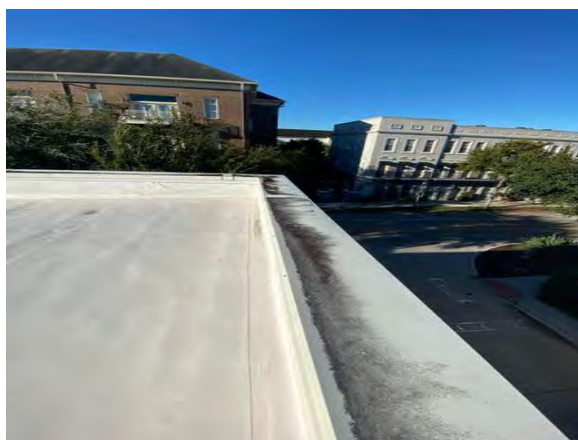
Front of building coping metal seems secure and watertight.
