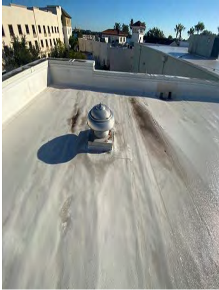
Curb flashing is secure and intact.
