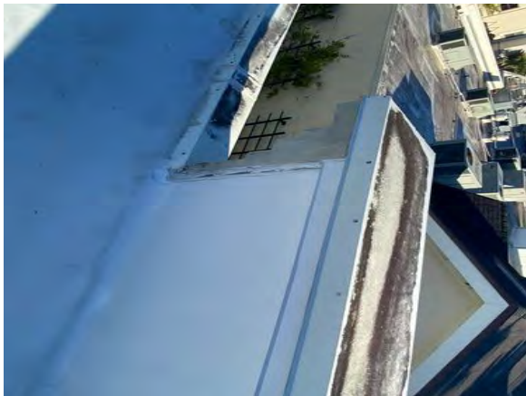
Metal flashing is watertight and secure
