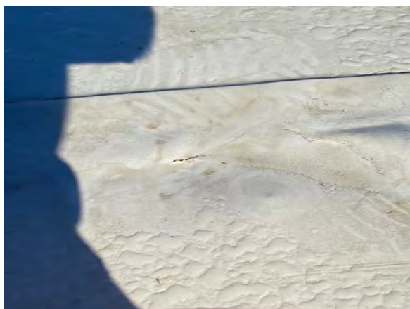
Possible opening in the future not all the way through.
