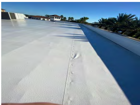
Example of roof seams.
