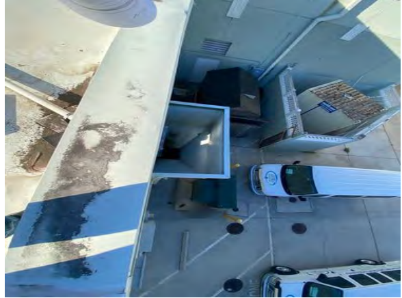
Down spout is clear from debris
