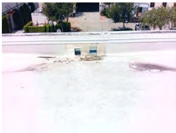
Overview of scuppers.
