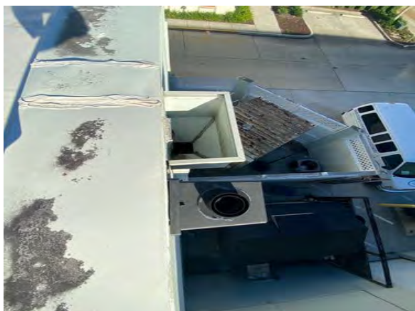
Down spout is clear from debris
