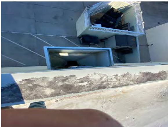
Clear from debris
