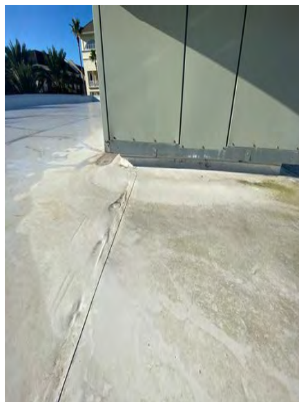
Example of curb flashing is secure and intact.
