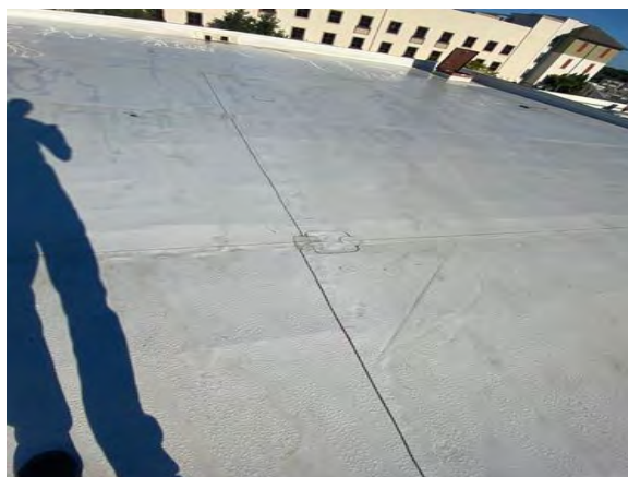
Overview of membrane and seams tight.
