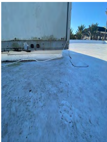
Curb flashing is secure and intact
